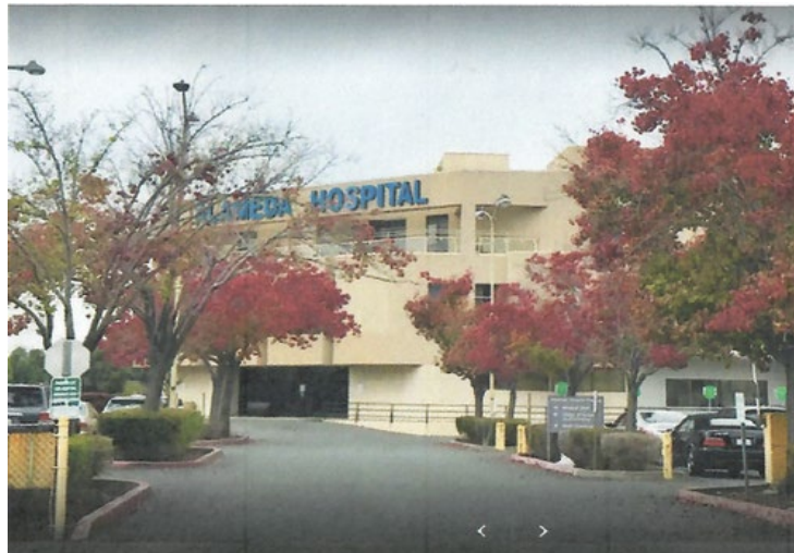
South Wing- Alameda Hospital
